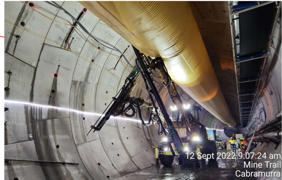
CT07 - Jumbo Install 6m rock bolts
