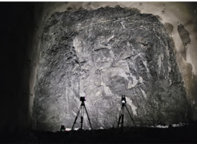
Fig. 2: MHC-face at S2.0257. Joints, minor tectonic faulting and bedding planes with minor deformations are visible. The tripods devices are photographing and laser scanning the exposed surface of the cutting. The contractor's geologist (and sometimes the S&L's technical team) are mapping the geology and rating the stability.
